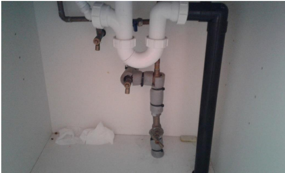
Internal Stop-Tap under kitchen unit
